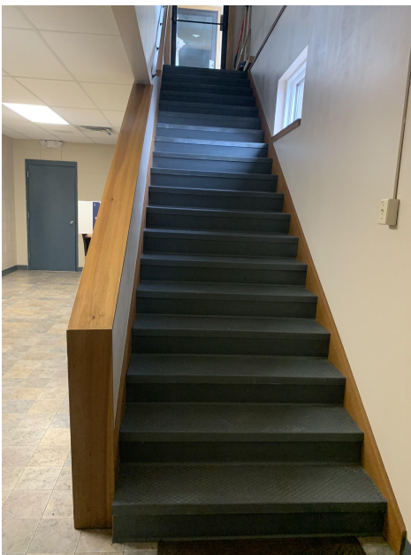
(H) stairs going to the basement.
