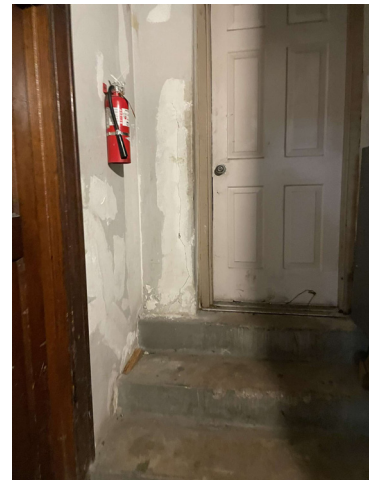
16 - Patched paint on wall
