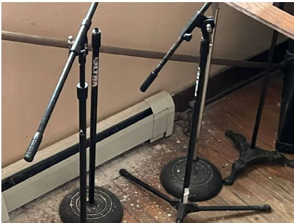
24 - Water damage in storage area
