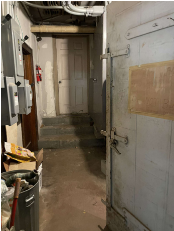
36 - Boiler room entrance
