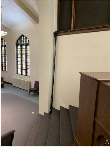
43 - Cords going down wall
