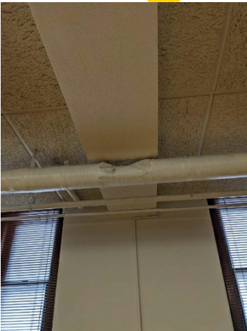
4 - Damaged pipe
