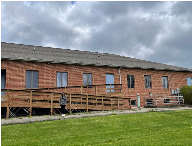
Rear side of building - has a ramp for wheelchair accessibility
