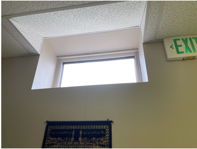
Clerestory windows throughout basement
