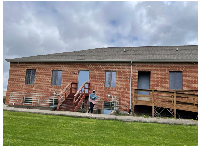
Rear side of building (West side)
