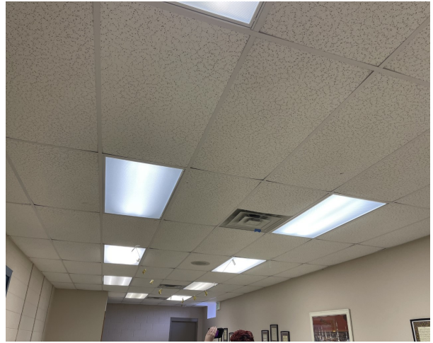
Ceiling in portion of multi-purpose room
