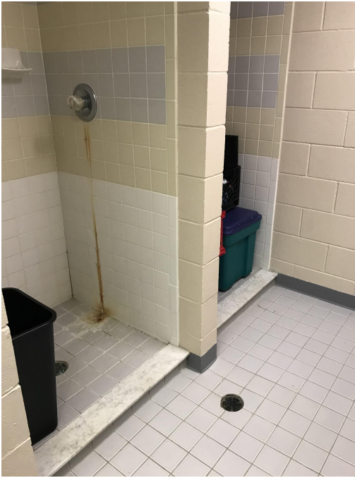
Showers in downstairs bathroom/sauna
