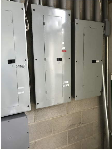
Breaker Panels downstairs - easily accessible to anyone (not good)
