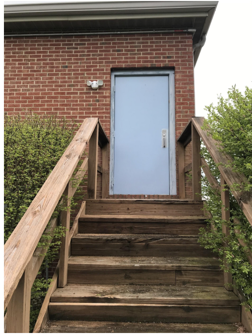
View of multiple rear entrances
